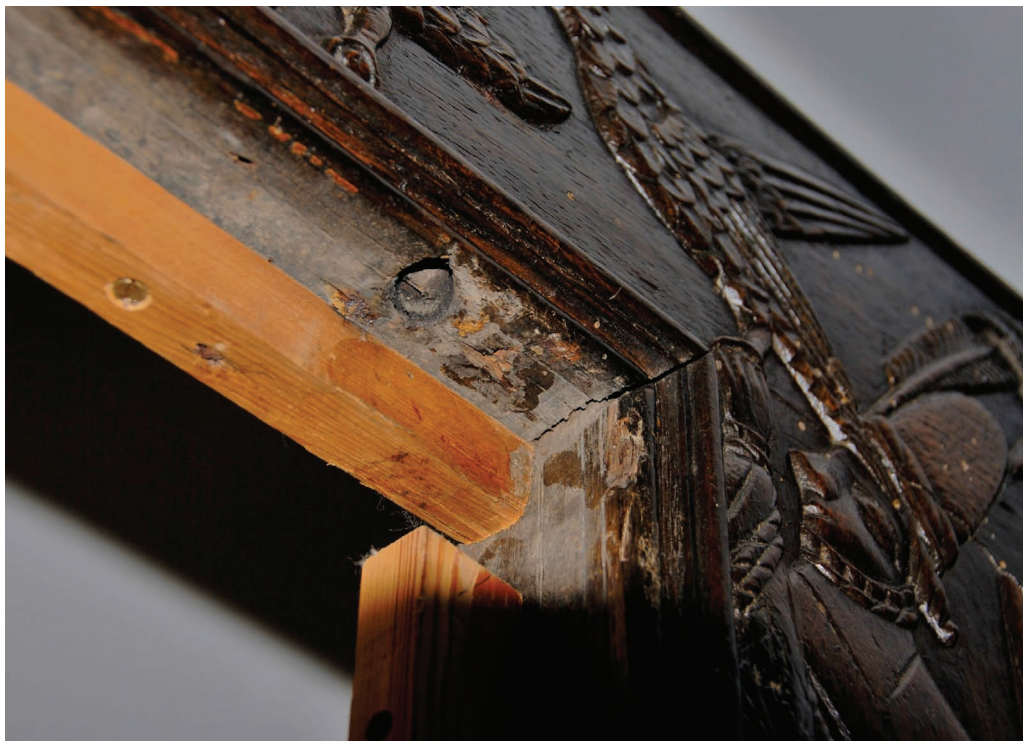
10 Cotehele cupboard, detail, showing the large diameter socket for a wooden pintle hinge. The author
