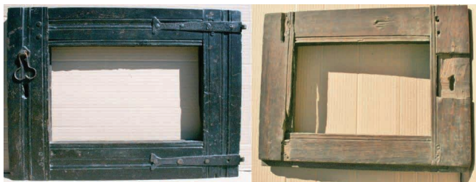
13 Two views of the upper right door frame, showing run-through scratch stock mouldings on the stiles, and on the inside faces of the stiles and rails. The author
