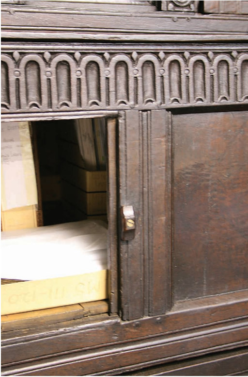
22 Two views of the left middle tier door and aperture, showing the shelf overlapping the front rail and (right) the rebate cut out of the lower edge of the door. The author
