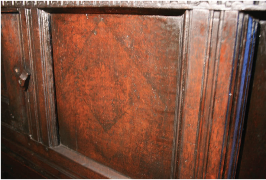
33 One of the lower panels, showing the outline of the original applied lozenge moulding. The author
