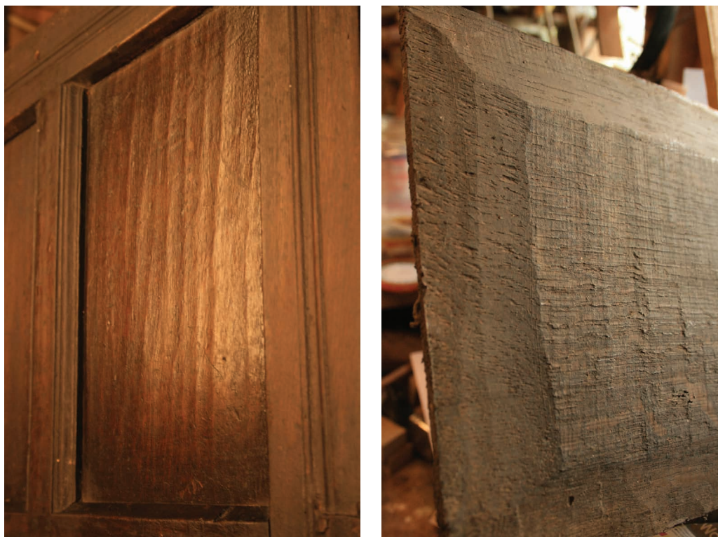
11 Two views of the press's panels, showing plane marks on the outside (left) and inside (right) faces. The author
