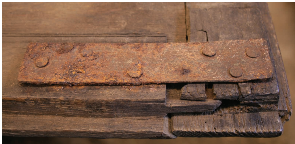
23 Inside face of the left middle tier door, showing how the joint has been weakened by the rebate cut in its lower edge, and the iron plate used to strengthen it. The author
