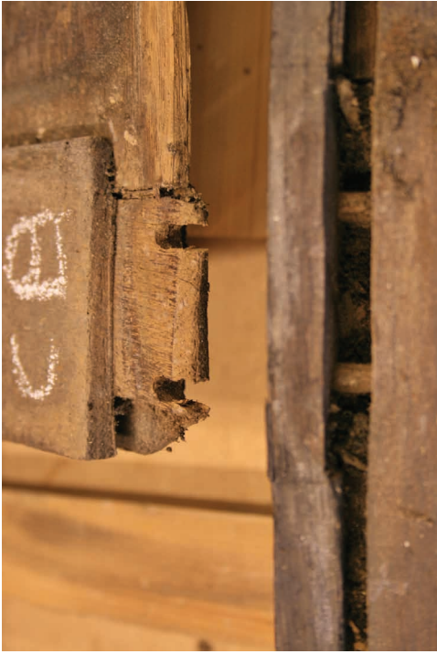
14 Dismantled joint, showing how the pegs have pulled through the short tenons. Note that the setting-out lines for the mortise are scribed to the full width of the rail rather than to the narrower tenon. The author
