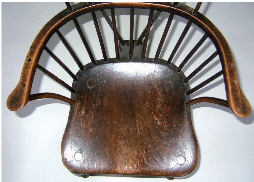
5 View of arm-bow showing tops of through-mortised spindles. John Boram
