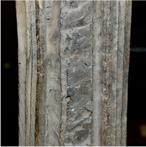
30 (above) Detail of muntin showing burlled timber, from parclose screen, oak, early sixteenth century, St Bartholomew, Bow, Crediton, Devon
