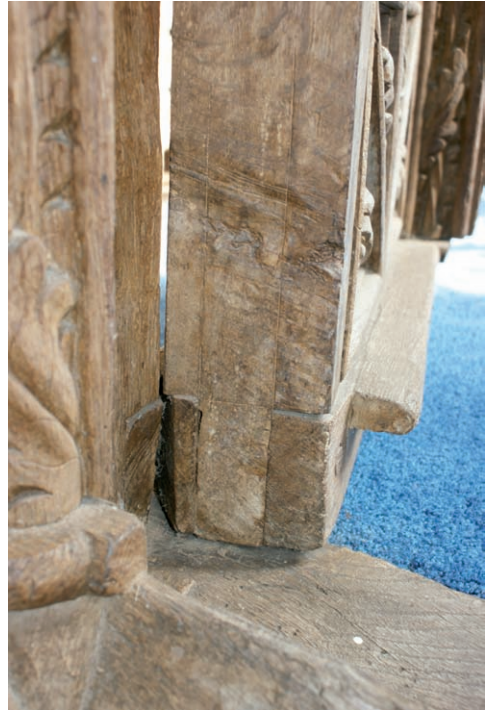
45 Detail of exposed tenon, from door framing of Rood screen, oak, early sixteenth century, St Matthew, Coldridge, Crediton, Devon
