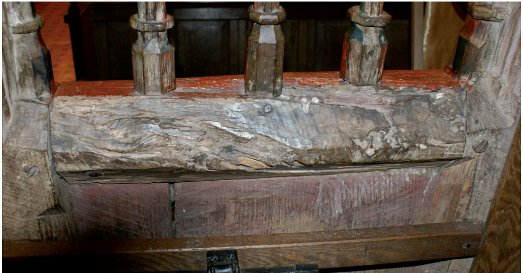
29 Detail of framing of dado showing poor quality timber, from reverse of Rood screen, oak, early sixteenth century, St Bartholomew, Bow, Crediton, Devon
