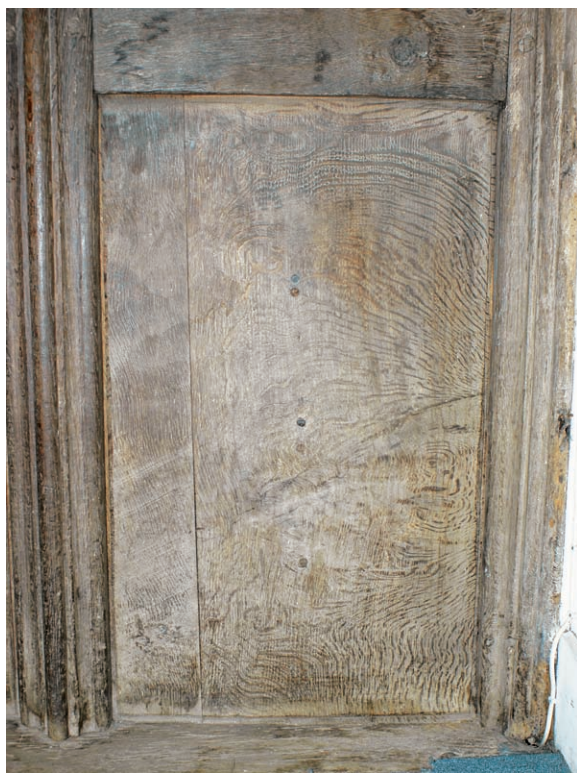
26 Detail of reverse of dado panel showing high-quality timber, from Rood screen, oak, c. 1540, St Thomas of Canterbury, Lapford, Crediton, Devon
