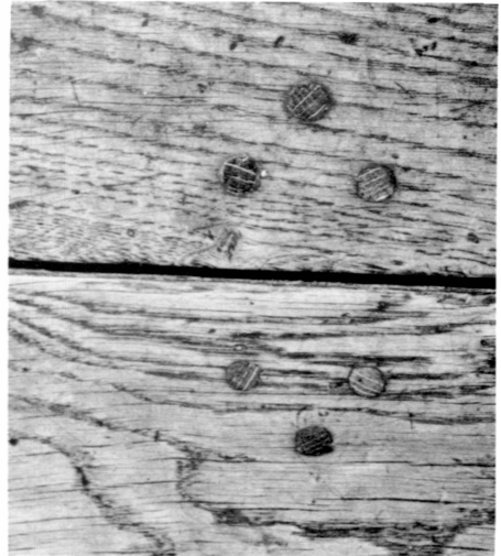
4. Detail of a pegged cross-tongue joint
