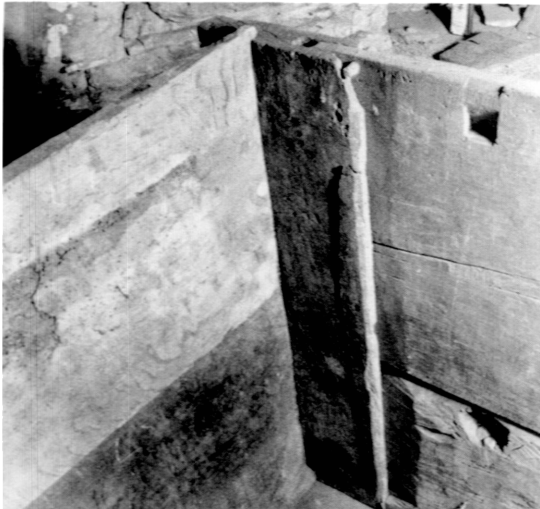
3. Detail of Figure 2 showing chamfered planks grooved into the stile, and one recess for a hook-rail hinge
