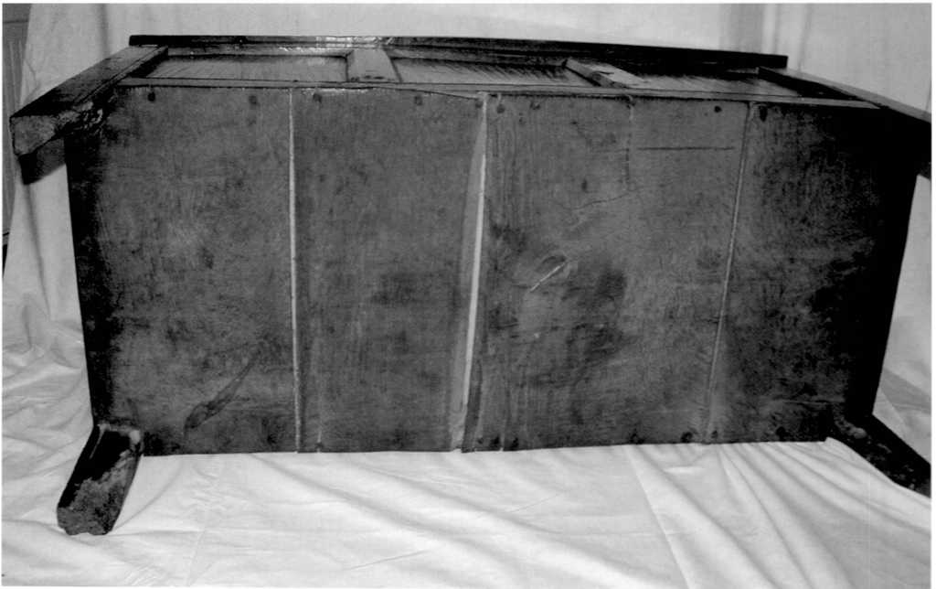
6. Base planks fixed from front to back
