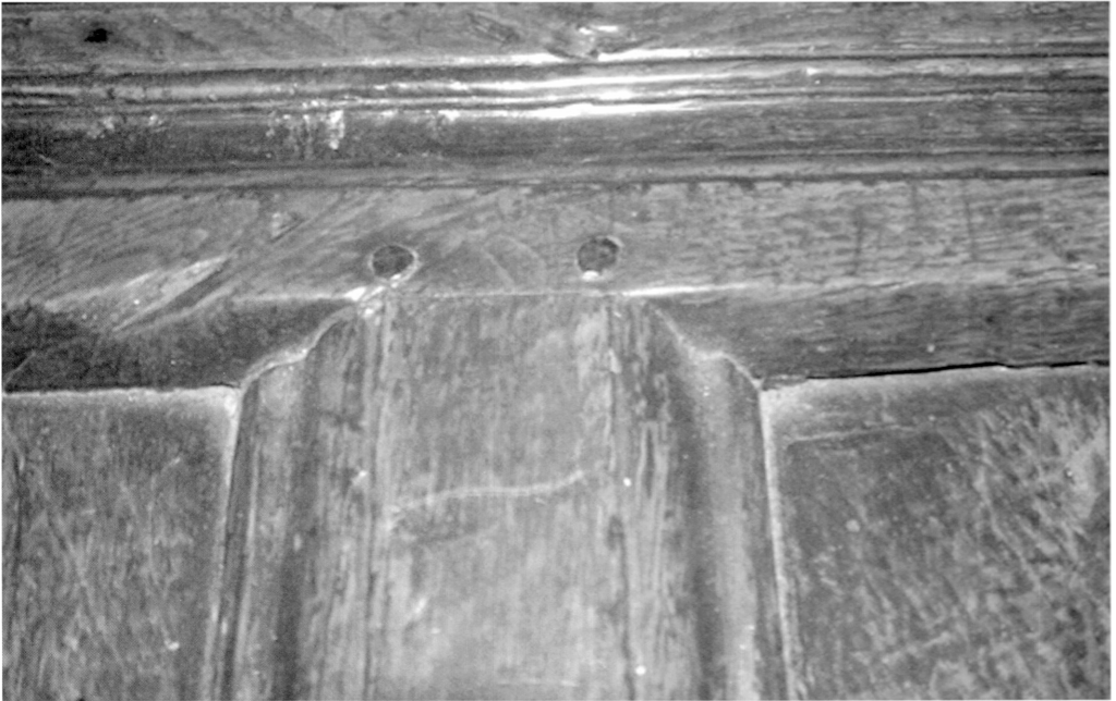
5. Pegs driven through the joint unions and channel moulded framed panels
