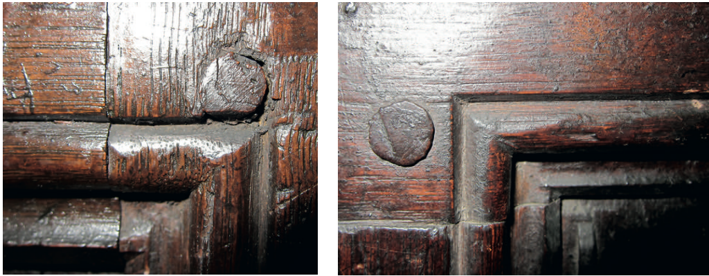
10 and 11 Details of panel framing at King's College Chapel, Aberdeen, 1506, showing distinctive profile of 30 mm-wide mouldings and large pegs.
