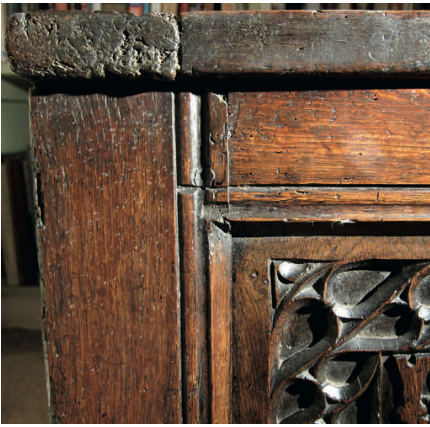
5 Full-length run-moulding of stile. The author
