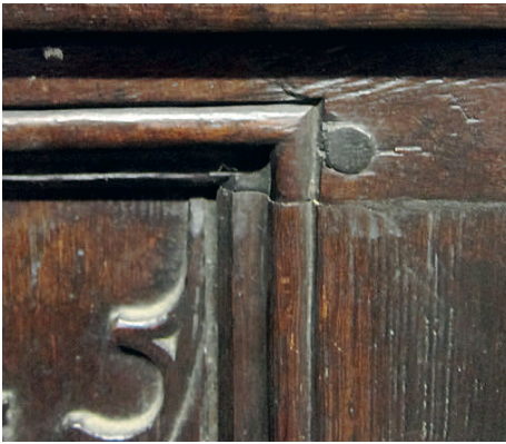
12 30 mm wide moulding and large pegs in panelling at St Nicholas' Kirk, Aberdeen, 1507. Courtesy St Nicholas' Kirk, Aberdeen: the author
