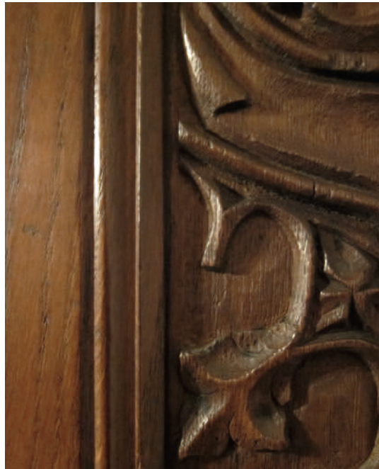
12 30 mm wide moulding and large pegs in panelling at St Nicholas' Kirk, Aberdeen, 1507. Courtesy St Nicholas' Kirk, Aberdeen: the author
