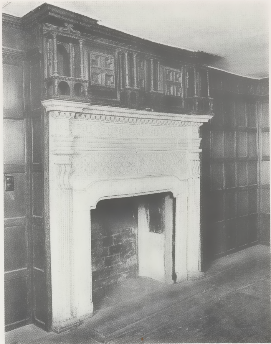
Fig. 1 Interior of the Merchant's House, Marlborough
