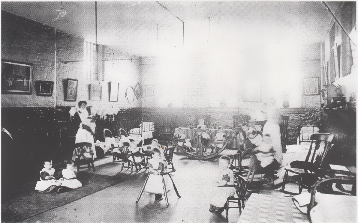
Fig 1. The Children's wing of the workhouse
