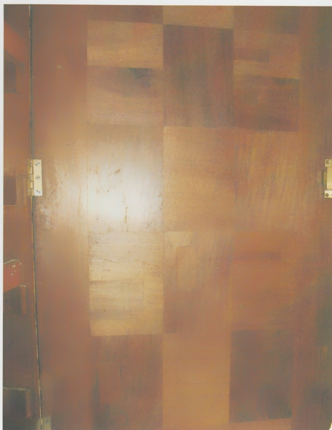
Fig 18 Inside view of the door showing block-panel construction
