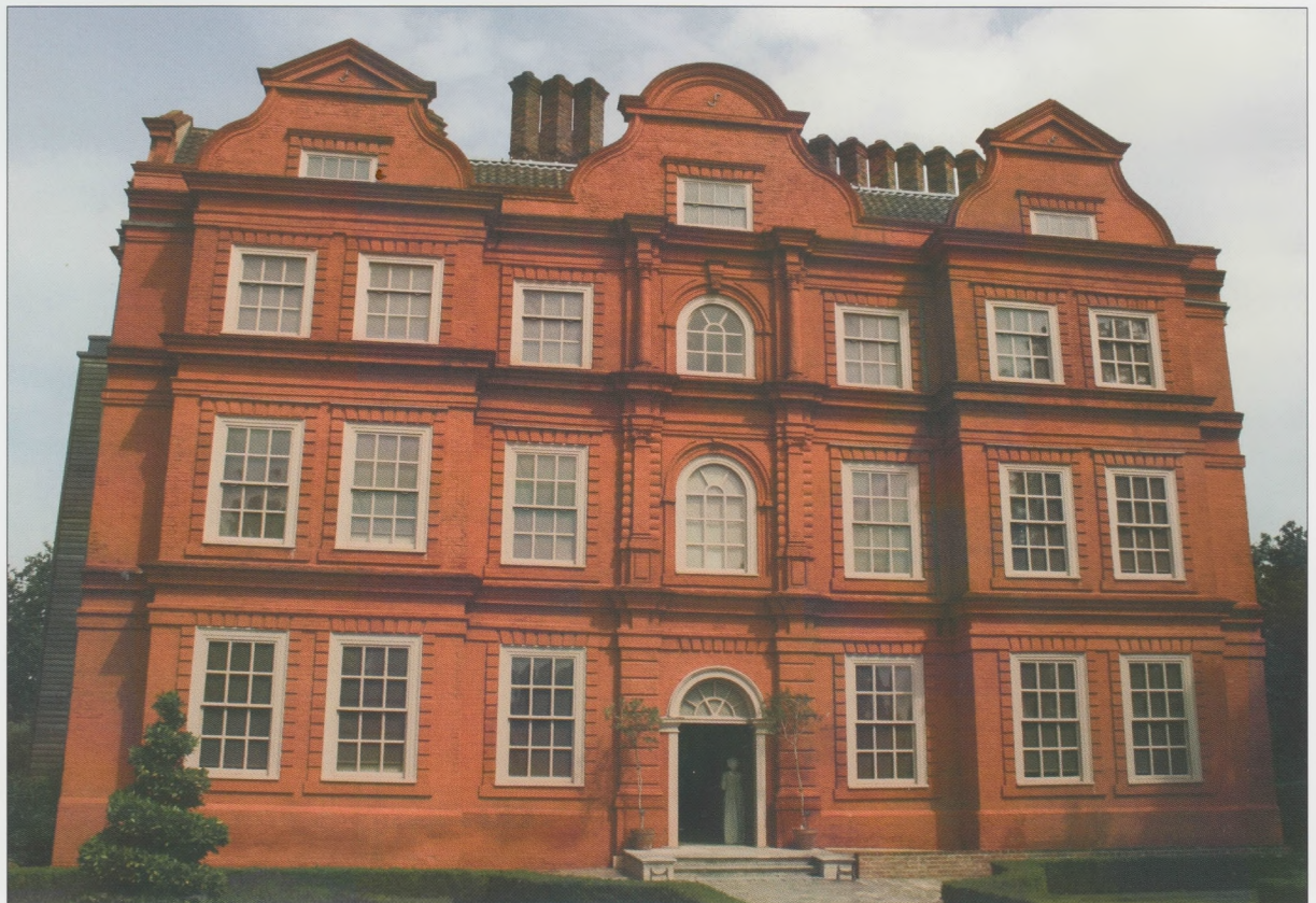
The painted brick facade of Kew Palace.
