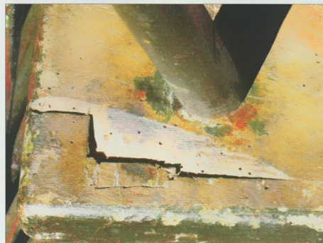
Fig. 4 The wany edge of the middle board
