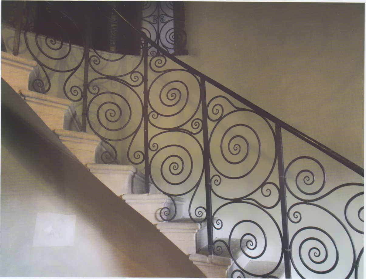
Fine wrought iron secondary staircase, late 17th century. It was not unusual to have a wrought iron stair balustrade for the secondary staircase of Scottish houses but this is possibly the earliest in date. (Courtesy of the National Trust for Scotland)
