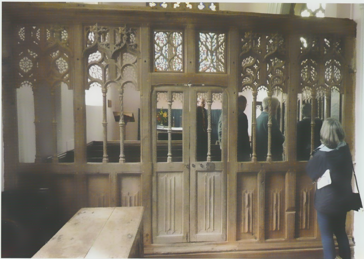
Fig. 1 St Andrew's, Colebrook, Devon. The five-bay rood screen; note the linen-fold panels
