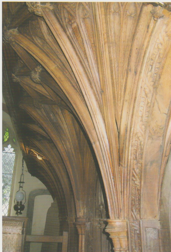
Fig. 11 St Mathew, Coldridge, Devon. The oak ribs of the rood screen
