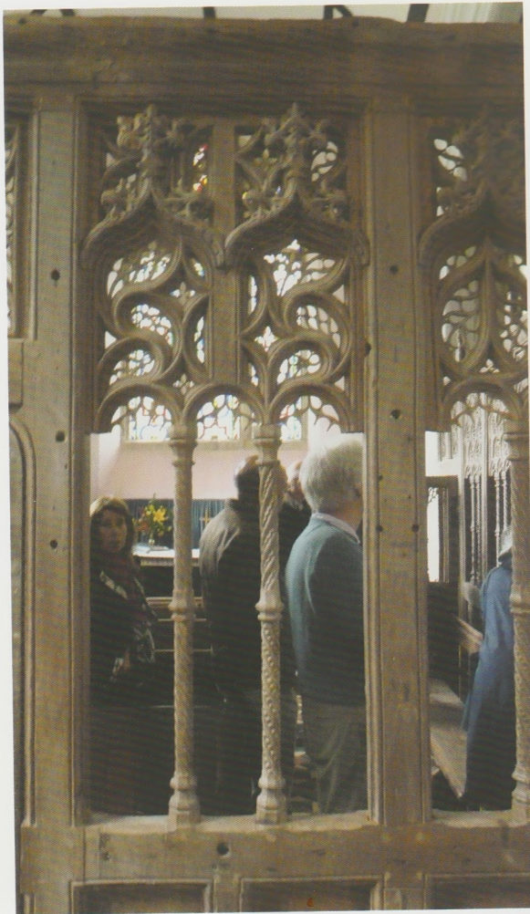
Fig. 2. St Andrew's, Colebrook, Devon. Note the holes in the uprights onto which carvings were fixed
