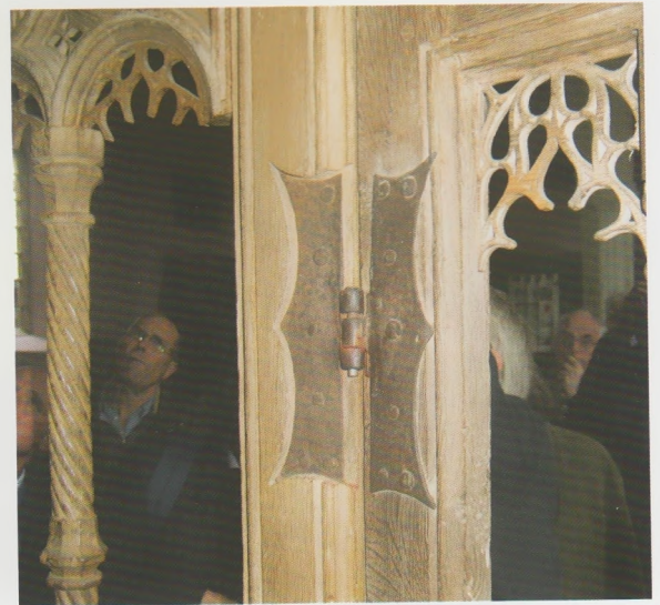
Fig. 4 St Andrew's, Colebrook, Devon. French style wrought-iron butterfly hinge
