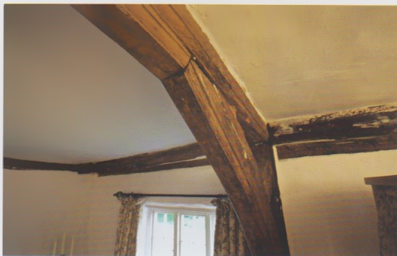
Fig. 4 The massive 14th-century oak roof brace in one of the upper rooms, Chaldon Court, Surrey
