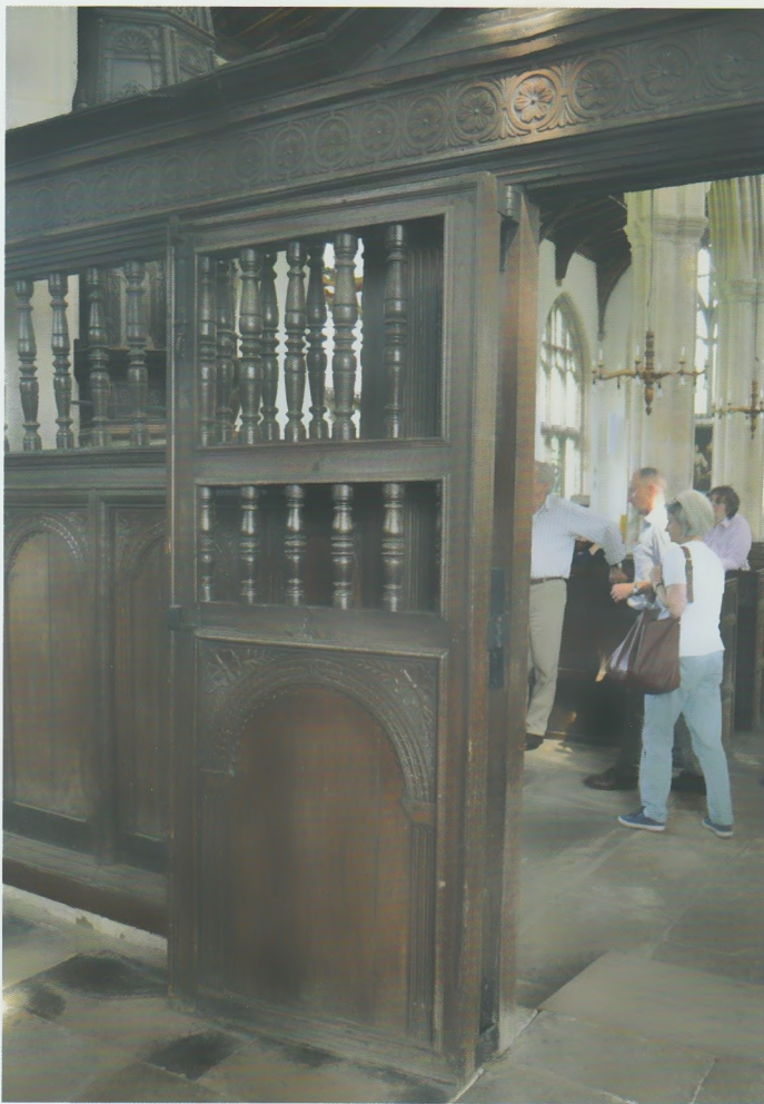
Fig. 16 The western screen of turned and carved oak that divides the church and which dates to c. 1630
