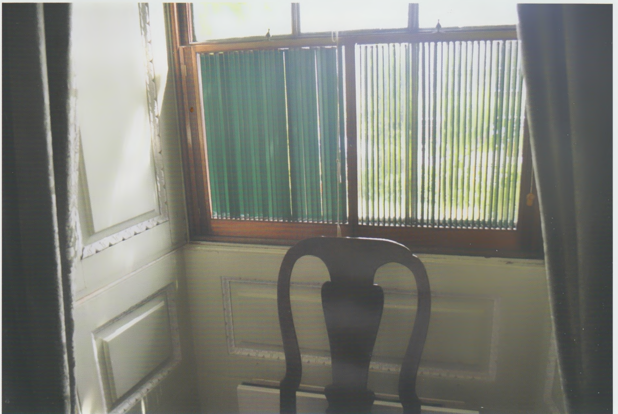
Fig. 14 A pair dwarf blinds, incorrectly and irritatingly termed 'snob screens' in the guidebook. It is possible to see from this picture how the vertical slats can be moved to alter the direction of the light
