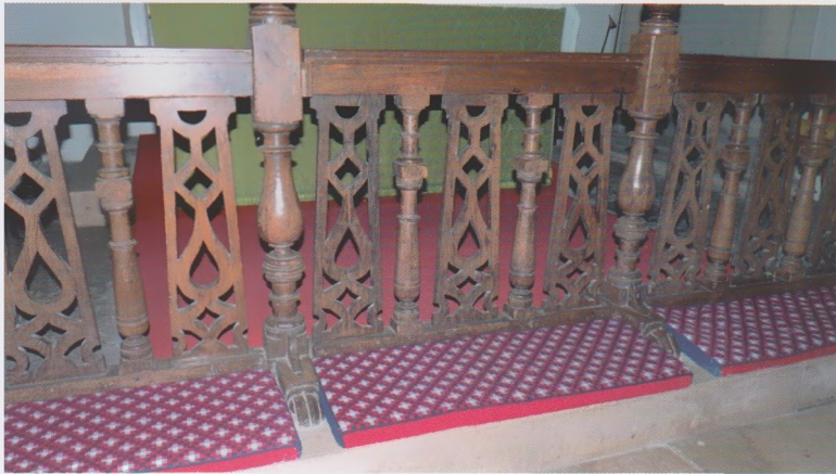
Fig. 9 St Andrew, Great Durnford, Wiltshire. The splendid turned and fretted-out oak communion rail
