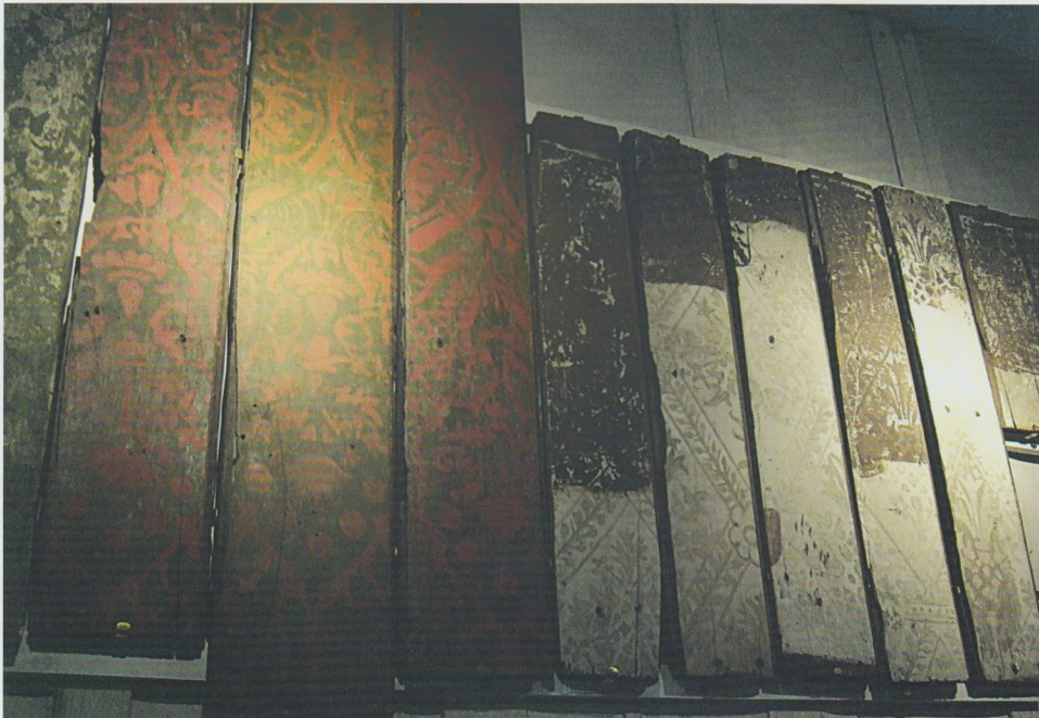
Fig. 6 Painted detail on the underneath of the floorboards
