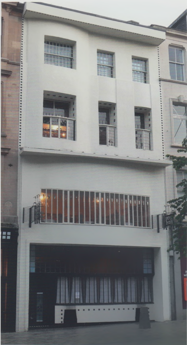
The restored exterior showing the large bay window of the Salon de Luxe on the first floor, now back in its original recessed position. (Photo Peter Jefferies)
