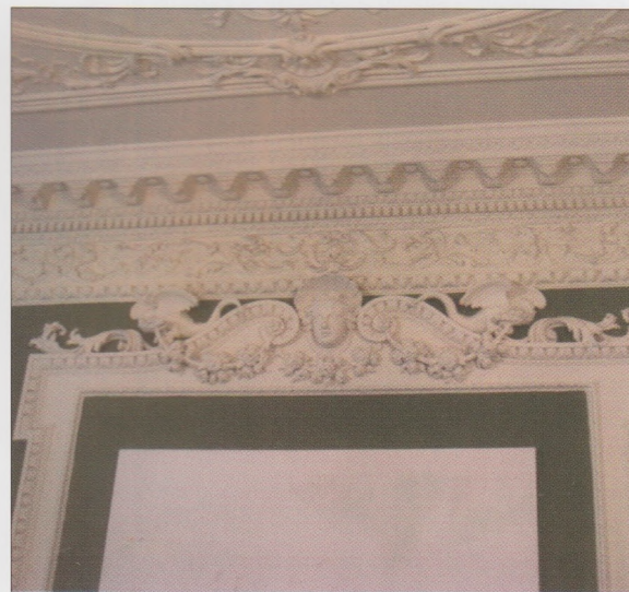
Plasterwork example at the House of St Barnabas
