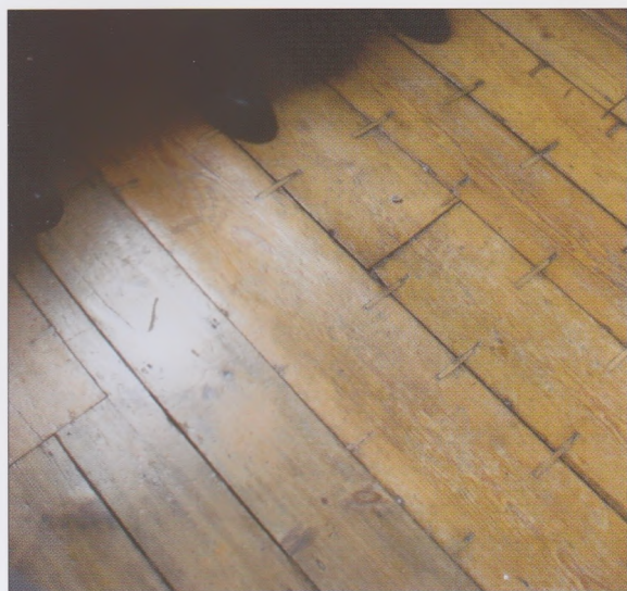
Boards worn down to show floor pegs.
