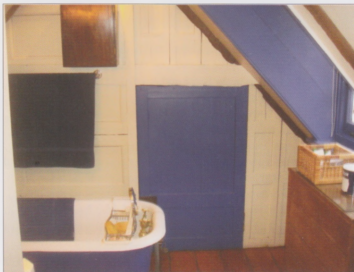
Attic room with shutter partition and four foot door
