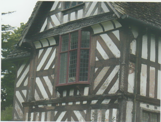
Timber-framing at Pitchford Hall, built from 1473. Photo Christopher Claxton Stevens
