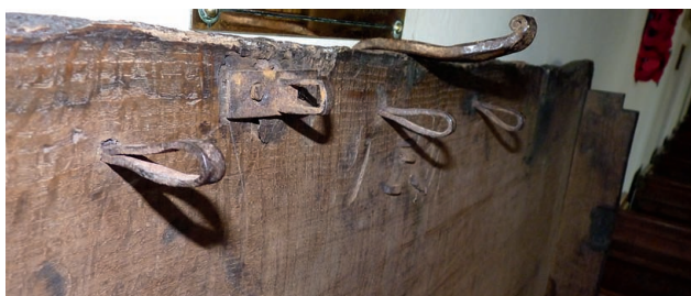
17 Stedham, staples on lid for sliding bolt lock. The Author
