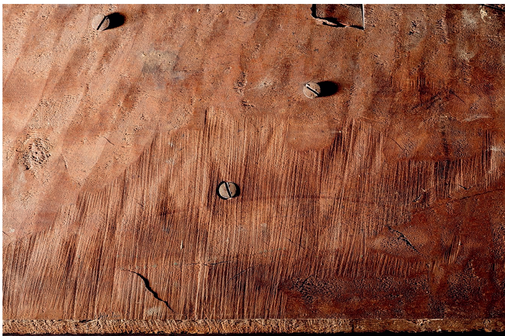
23 Characteristic marks made by a pit saw on the back of the crenellated gable. Sam Noonan
