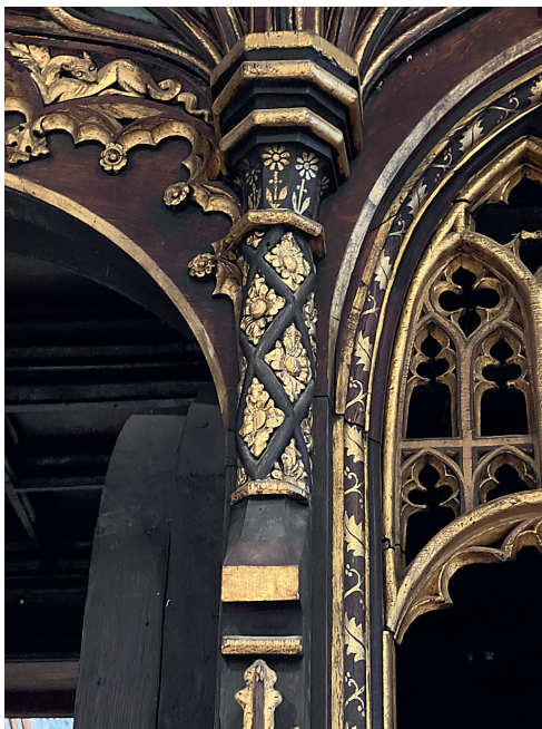
12 Detail of the Diaper-Work on the pulpitum, Manchester Cathedral, 1520s. The author
