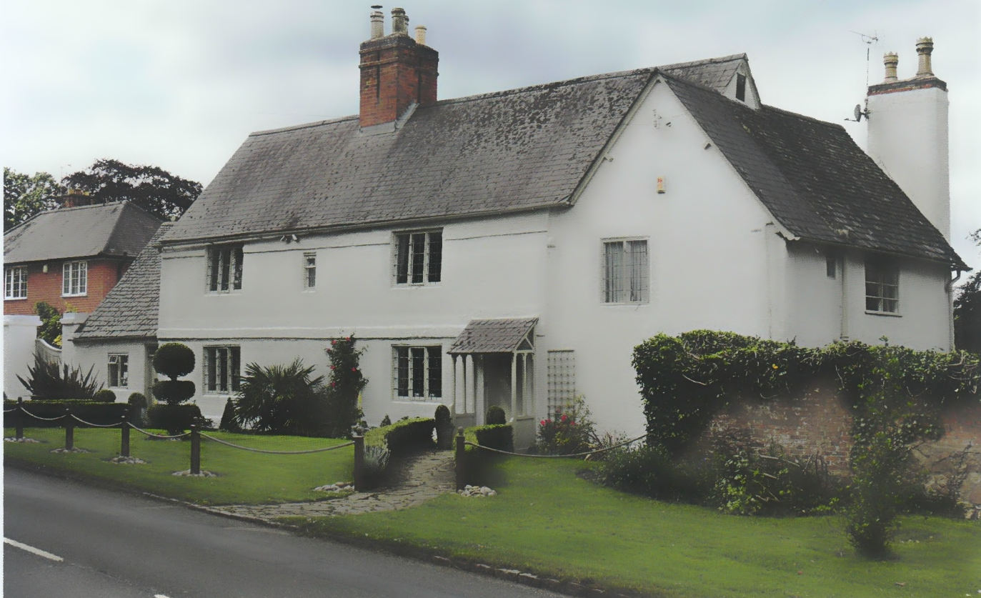
A house in the main street in Cossington, Leicestershire which has the same hall-and-cross-wing plan form as the house of John Oswin the weaver. At the left-hand end a single-storey unit could perhaps have been a loom shop. Photo Linda Hall
